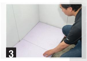
Install the first row of panels until you reach the end of that row, trimming the last panel to fit. If the resulting cut-off is greater than 18" long, you can use it to start the next run of panels. Make sure you install shims between the DRICORE Insul-Armor panels and the finished walls, so panels don't shift during installation.. Some installers prefer taping the joints of the panels with a vapor barrier rated tape to help hold the panels in the first 1-2 rows together during installation.
