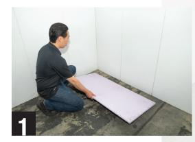
While you can lay the DRICORE Insul-Armor panels in either direction, it is generally laid with the 4' length running the longest dimension of the room.
