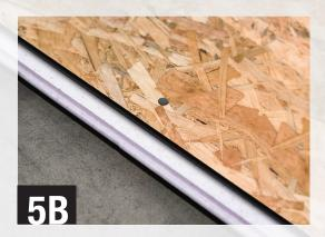
Screw down each panel of OSB, plywood or any other substrate used. Depending on the thickness of the substrate chosen, screws must penetrate the concrete a minimum 3/4". DRICORE Insul-Armor is 1" in thickness, therefore, a 3/8" substrate would require a nail no shorter than 2 1/4" in length.
