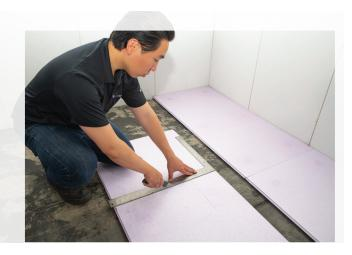
In the event that damage does happen to the DRICORE Insul-Armor panels after being installed, simply cut out the damaged area, replace with a fitted piece matching the cutout dimensions, and tape the seams using a vapor barrier rated tape (available at buidling supply stores in the vapor barrier section).
