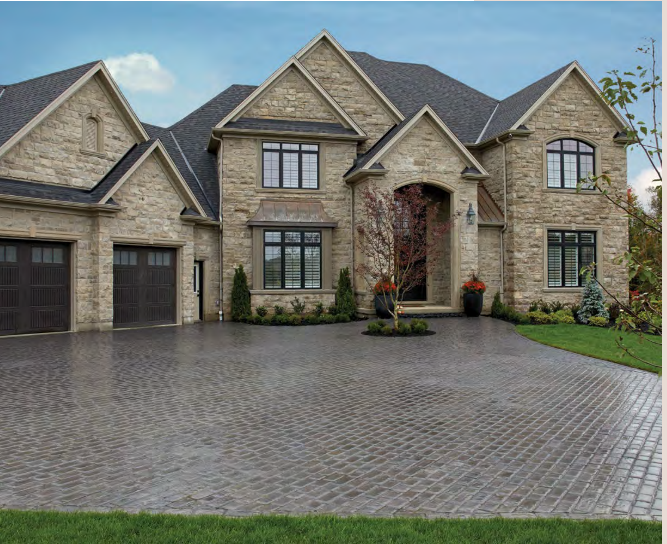
Pavers: Enviro Passagio, Mountain & Salem blended on site (shown wet)
